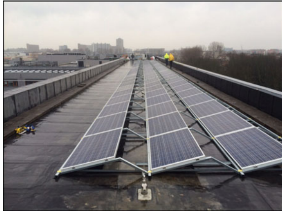
Fig. 4 Installation of solar energy on campus buildings. Source TU Delft
