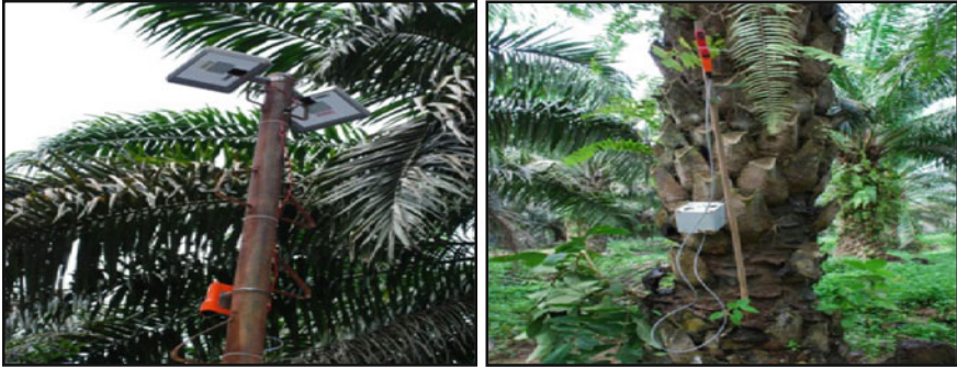
(a) Gateway installation - fixed pole and powered by car battery & solar.
