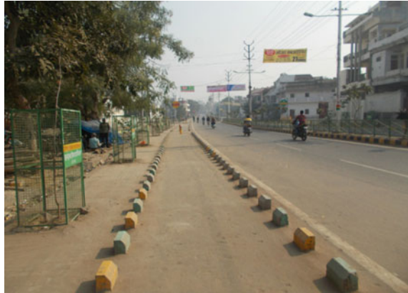
Fig. 8.5 Newly constructed road with wider footpath in Mumfordganj. Source Author
