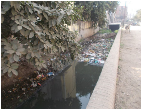
Fig. 8.8 Katra Nala and its roofing. Source Author
