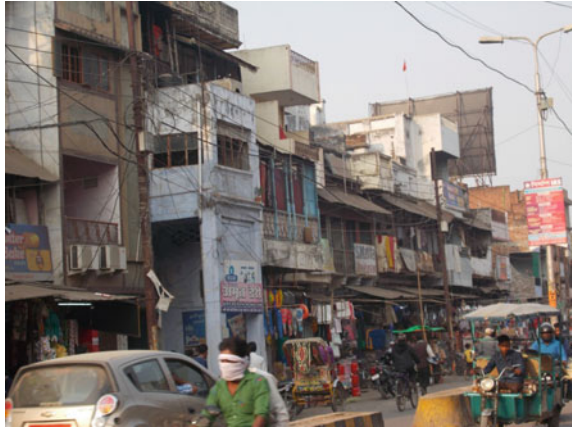
Fig. 8.1 Vulnerable residential buildings in Katra. Source Author
