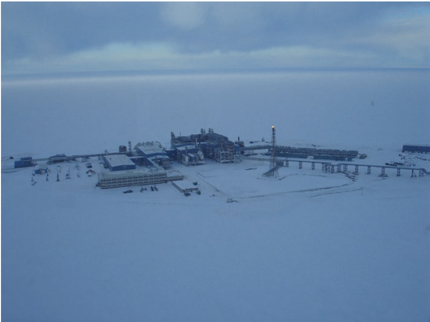
Fig. 24.4 Aerial view of an oil rig and infrastructure located in Prudhoe Bay, southern Beaufort Sea, Alaska. The oil rig is on an artificial island located approximately 8 km from the coast. A pipeline (right side of figure) runs from the rig to the mainland. Image credit: US Geological Survey
