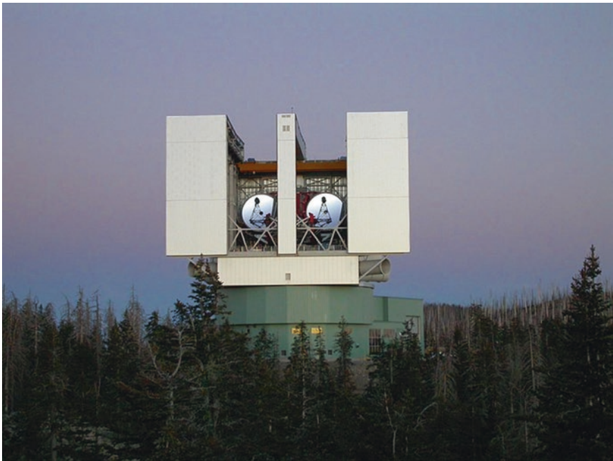
Fig. 5.69 The “King” of the Binoscopes! The LBT (Large Binocular Telescope) with its twin 8.4 M mirrors sits on Mt. Graham in Arizona. That is one big binocular telescope! (Image credit: NASA—Wikimedia Commons)
