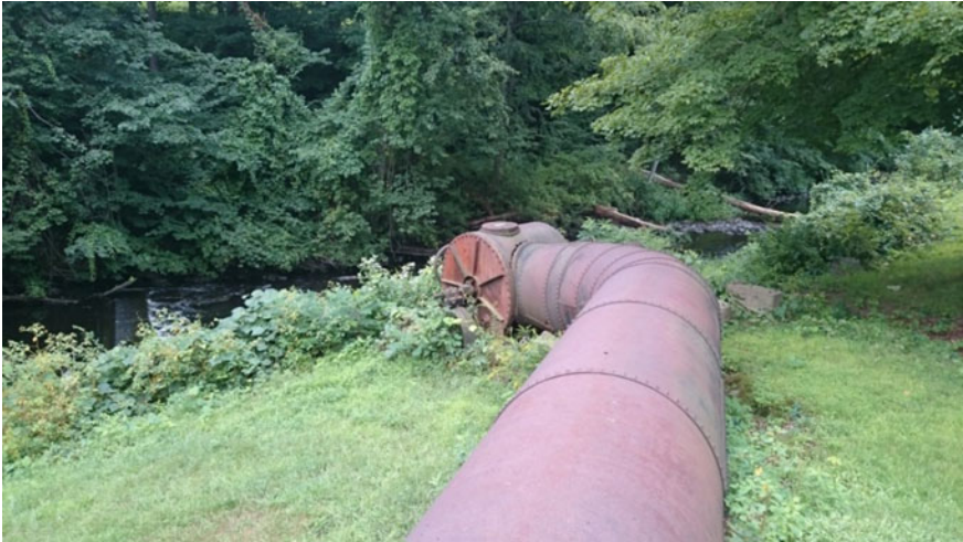
Fig. 3.1 A Penstock carrying water from a dam to power house to run hydraulic turbines. http://www.nebrownstone.com/blog/wp-content/uploads/2015/08/DSC_0019-1024x576.jpg
