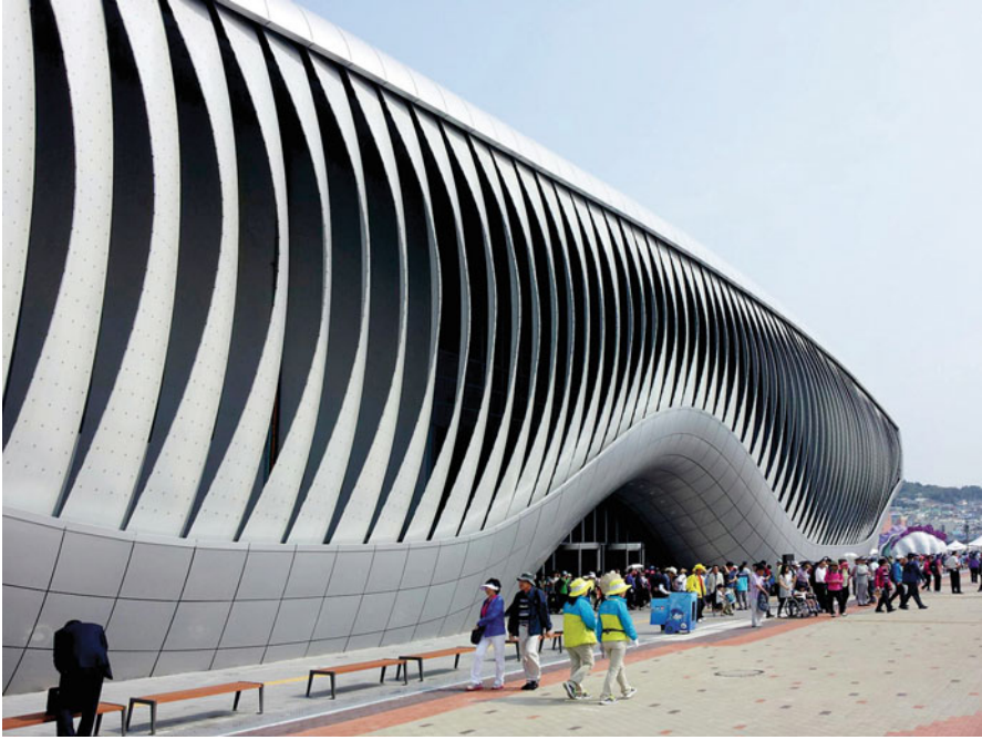
Fig. 3.6 “One Ocean”, building of the Expo 2012 in South Korea, is a masterpiece of bionics. The moving lamellae are based on the sophisticated opening mechanism of the bird-of-paradise flower ( Strelitzia ). The hinge-less flapping technology was developed by the groups around Jan Knippers and Thomas Speck and the kinetic facade was designed by the Austrian Soma architects and Knippers Helbig Engineering in Stuttgart. Even the hierarchical-structures composed of glass fiber reinforced polymer material for the kinetic façade are influenced by the hierarchical structured material from biological models (Photograph: Riccardo La Magna)
