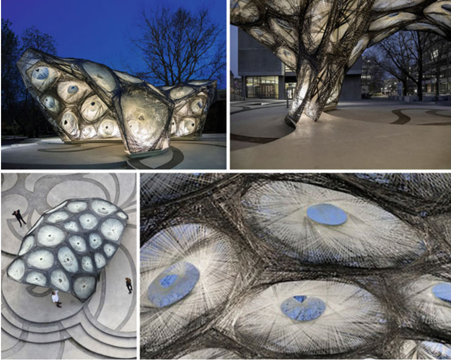
Fig. 4.7 ICD/ITKE Research Pavilion 2013–2014 (Dörstelmann et al. 2014; Parascho et al. 2014) inspired by fibre orientation around pores in insect cuticle. Courtesy of ICD and ITKE, Stuttgart, Germany
