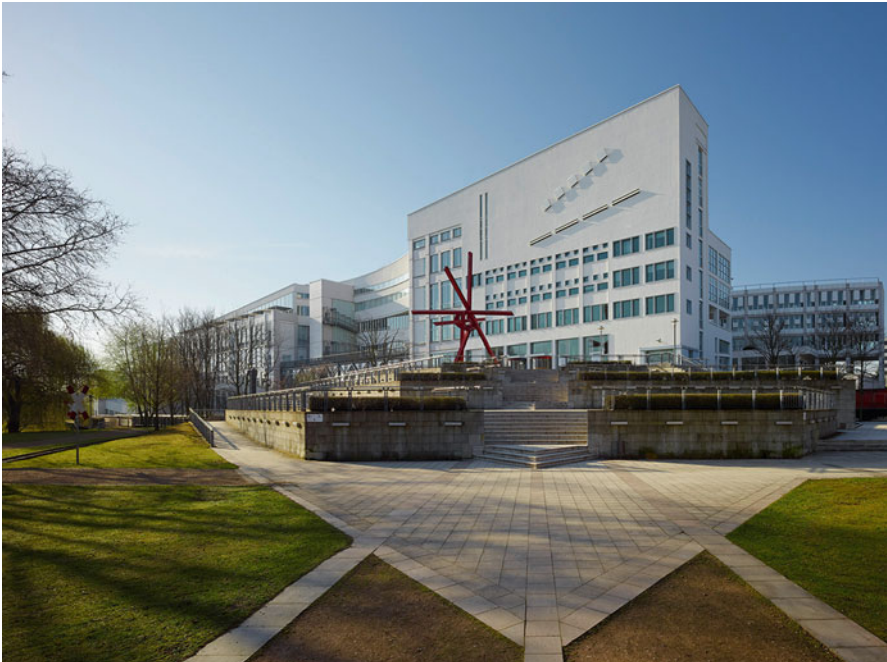
Fig. 3.12 Biomimetic architecture and sustainability: the Technoseum (a technical museum in Mannheim, Germany) has a self-cleaning Lotus-Effect® surface. The biomimetic coating is sustainable and lasts several decades – facades have to be repainted after this time. The conventional building itself may last more than a century. Time-limited sustainability is a principle of living prototypes: Lotus leaves last only for a short time span and are permanently renewed. Their rhizomes, however, may grow for centuries, and Lotus seeds may even germinate after more than 1200 years. Source: “Technoseum, zooey braun”
