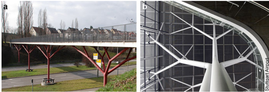
Fig. 10.2 Typical bifurcations in architecture (a) Pedestrian bridge, Pragsattel Stuttgart; (b) Branched column, Airport Stuttgart
