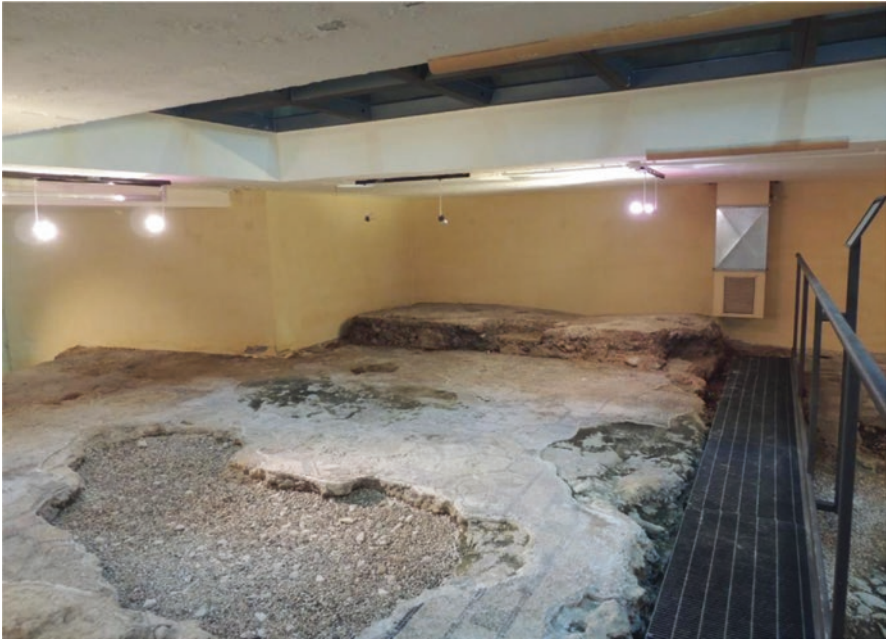
Fig. 2.1 Hypogeum archaeological site – in addition to the glass ceiling ( dark area at the top ) allowing natural light to penetrate, two older-generation lighting systems are visible: fluorescent tubes lacking UV guards and halogen spotlights generating considerable heat and relative air movement. This lighting system combined with high relative humidity levels increases the risk of biodegradation. The site is currently closed to the public
