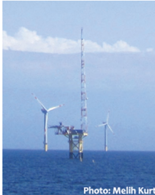
Fig. 5 Offshore research platform Fino1
