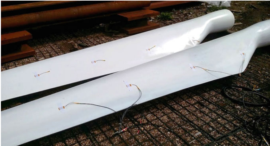
Fig. 5 Inspection of delamination in a wind turbine blade employing ultrasonic guided waves
