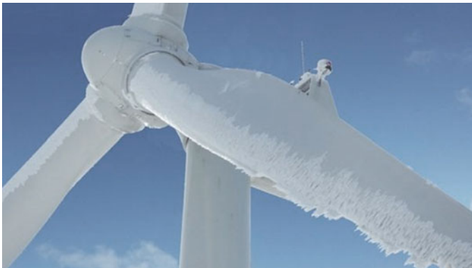
Fig. 2 Ice on the rotor of wind turbines
