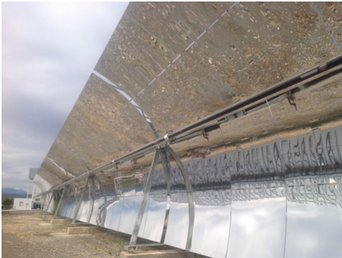
Fig. 1 Example of parabolic trough CSP technology at Plataforma Solar De Almeria (PSA) facility, Tabernas Desert, Spain
