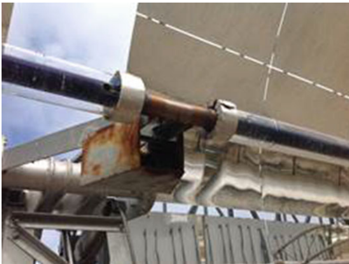
Fig. 6 Standard solar absorber tube and connection between two solar absorbed tubes
