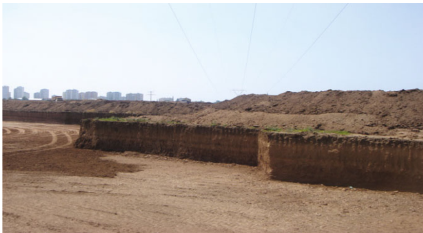
Fig. 10.1 The prime agricultural soil stripped for the construction of a building foundation, the Menzilat soil series. Source The authors
