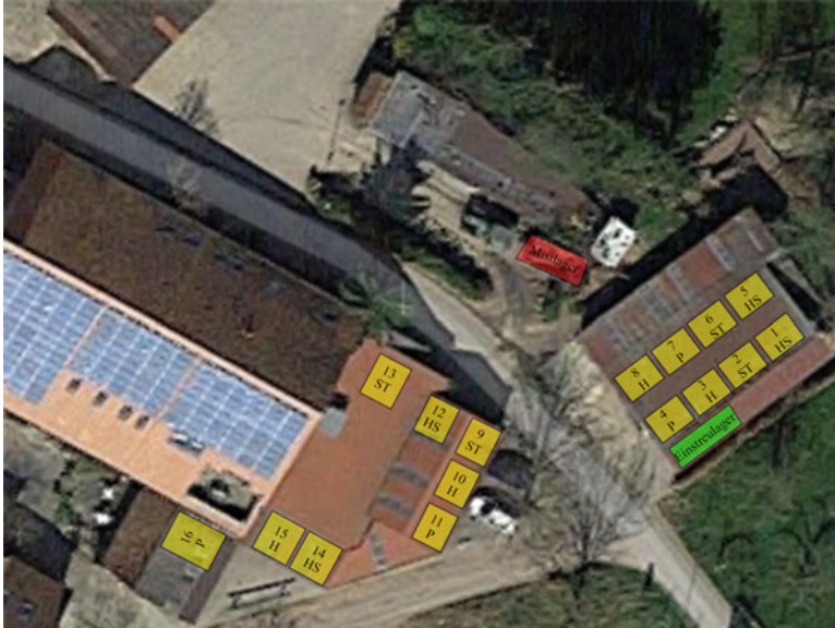
Fig. 24.1 Aerial view of the horse farm Reckerstal. Boxes are indicated in yellow with the following abbreviations for bedding material: ST straw, HS wood shavings, H miscanthus chips, P miscanthus pellets; Green area storage for bedding material; Red area manure storage. Source of photo: maps.google.com
