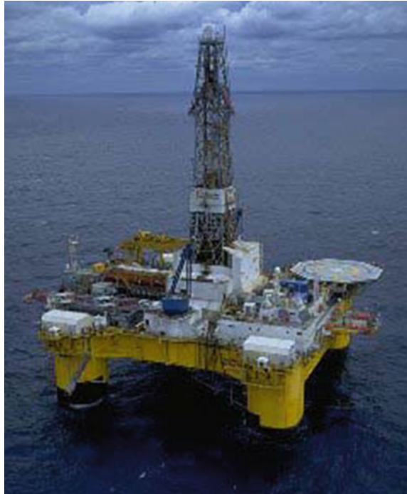
Fig. 7.10 A semi-submersible offshore platform (Source http://www.rigjobs.co.uk/oil/semisub.shtml )
