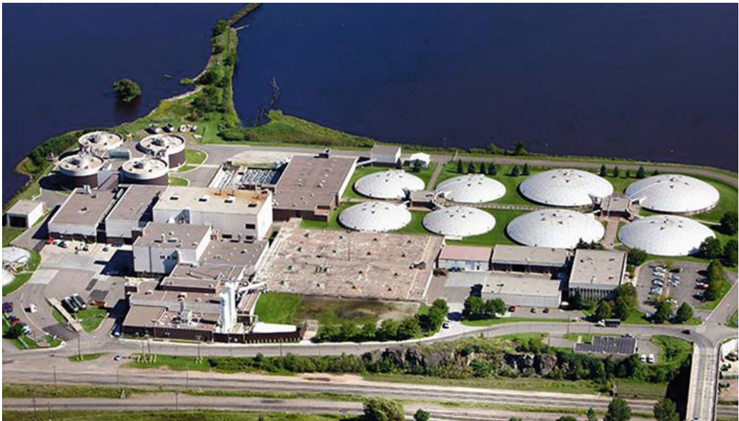
Fig. 12.8 Wastewater treatment plant on the shores of Western Lake Superior in Minnesota, USA. The Activated Sludge system is designed to treat 48 million gallons of wastewater per day (mgd) with a peak hydraulic capacity of 160 mgd. (Photo courtesy of Western Lake Superior Sanitary District.)
