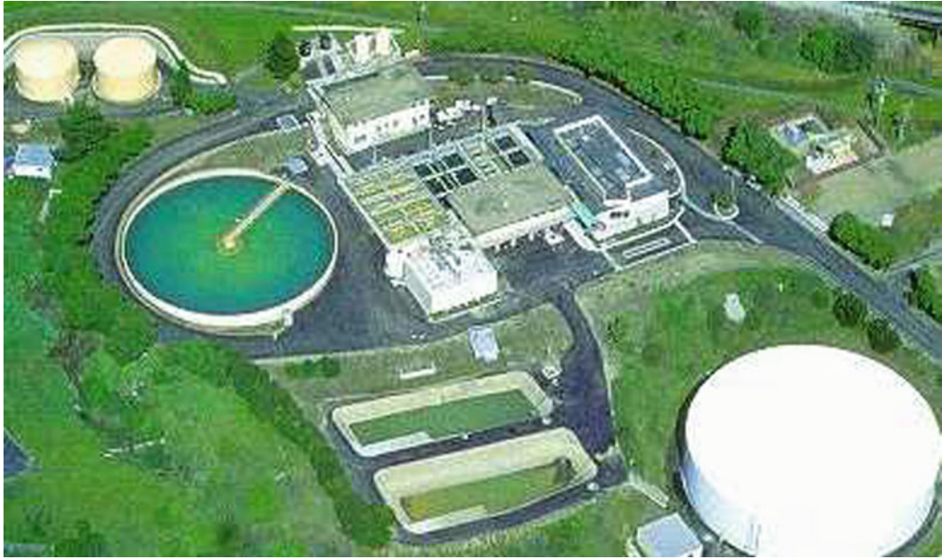
Fig. 12.3 A 6-million gallon per day water treatment plant at San Luis Obispo, located about halfway between Los Angeles and San Francisco on the Central Coast of California
