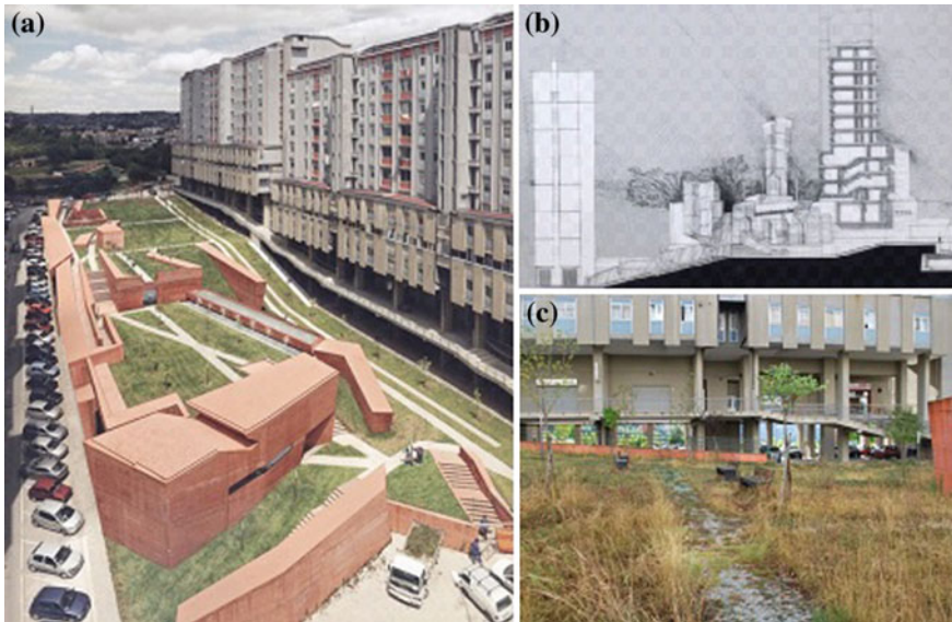
Fig. 10.2 a The realised project ( left ), b the original project ( right-up ), c the roof garden totally abandoned ( right-down ) (Source www.archea.it ; authors)
