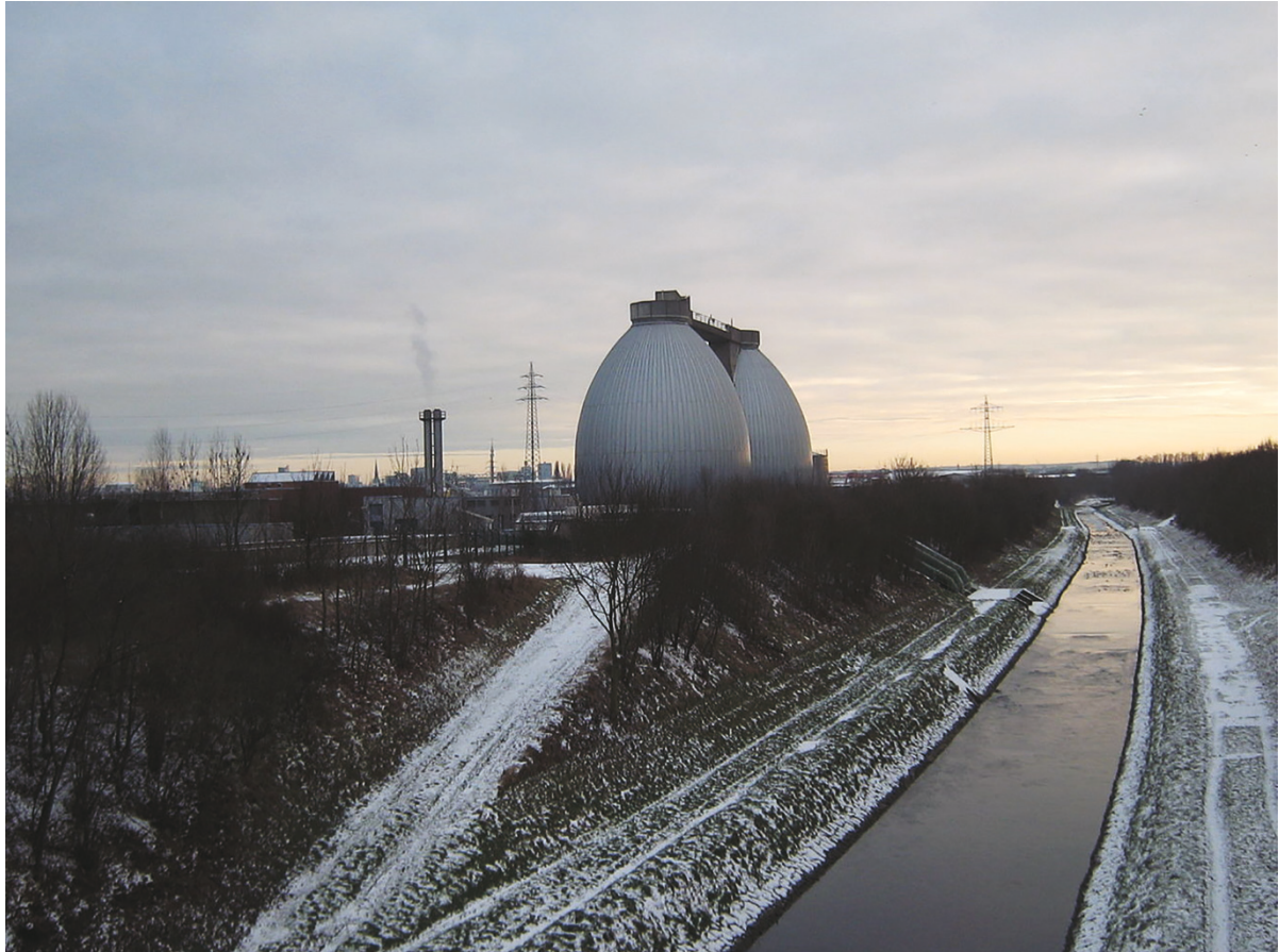
Figure 28.4: Wastewater treatment plant Deusen at the river Emscher. Source: Tbachner—Own work. Licensed under Creative Commons Attribution-ShareAlike 3.0 via Wikimedia Commons.
