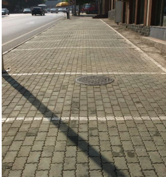
Fig. 3.12 Sidewalks have been taken over in Chinese Cities for on-street parking (Dalian) Photo by Jeffrey Kenworthy
