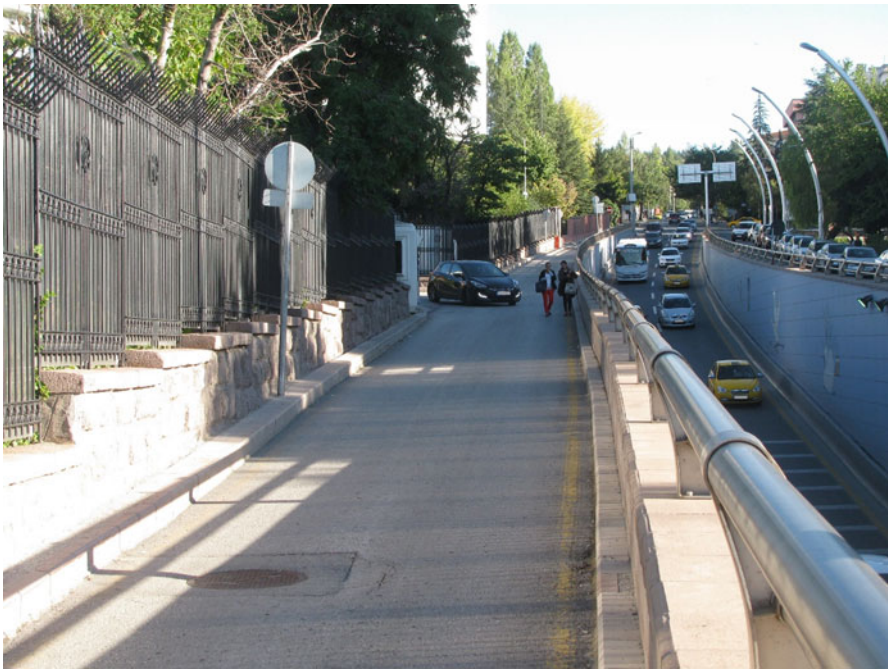
Fig. 12.6 Sidewalks narrowed to accommodate a tunnel in Ankara. Photo by author
