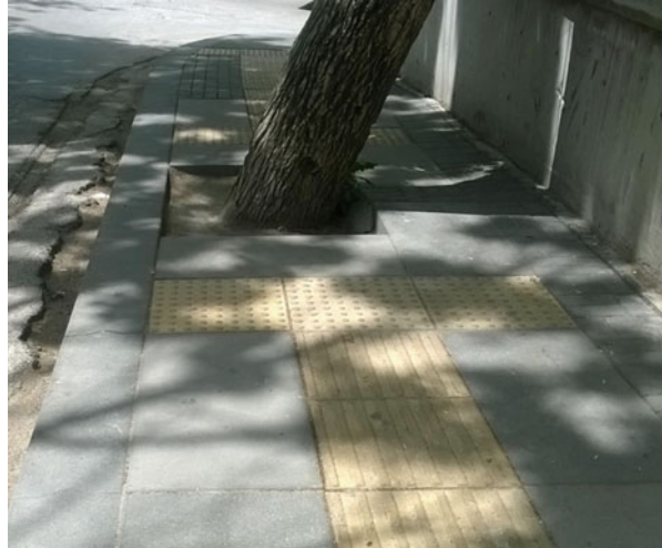
Fig. 12.5 Pedestrian and disabled access hampered by plantings on narrow sidewalks in Ankara. Photo by author
