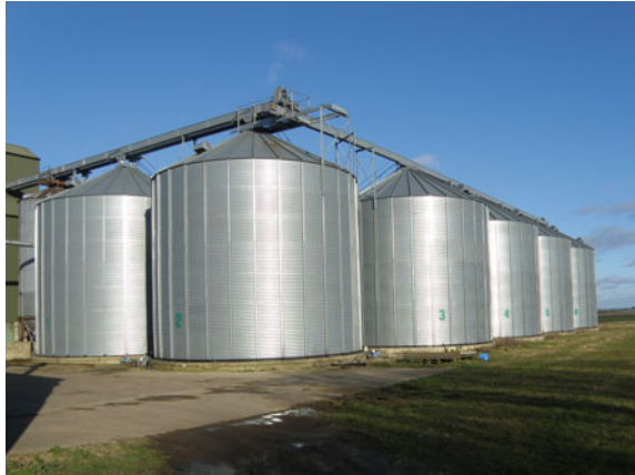
Fig. 2 Grains storage silo [7]
