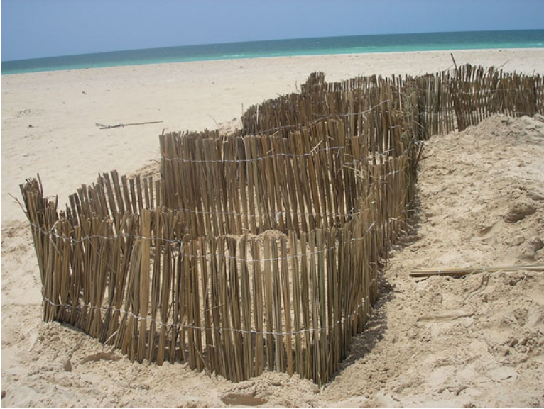
Fig. 19.8 Experience of sand dune stabilisation using Typha australis stalks on the dune between the “Plage des pêcheurs (Fishermen’s Beach)” and the wharf (Author’s own figure)
