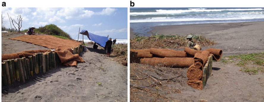
Fig. 20.8 Pictures of the on-site coir geotextile installation: (a). shows the cross-sectional view on the textiles; (b). shows the bamboo wall and the installation of the top coir layer © David 2014
