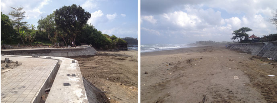
Fig. 20.6 Hard-structure seawall in Tabanan, Bali © David 2014
