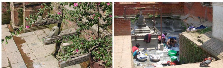
Fig. 15.2 Examples for stone spouts and their use by local communities (by author)
