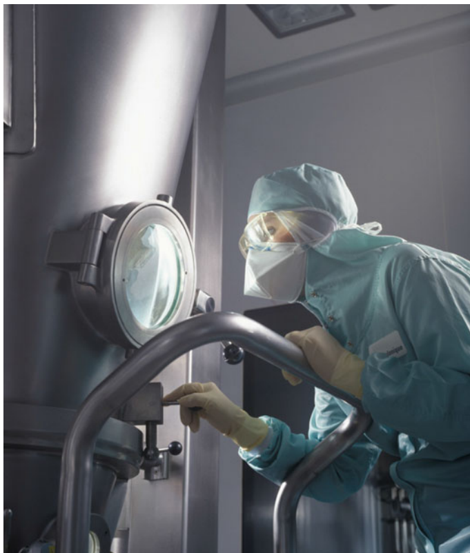
Fig. 2 A fluid-bed dryer being inspected during operation (Image courtesy of GlaxoSmithKline)
