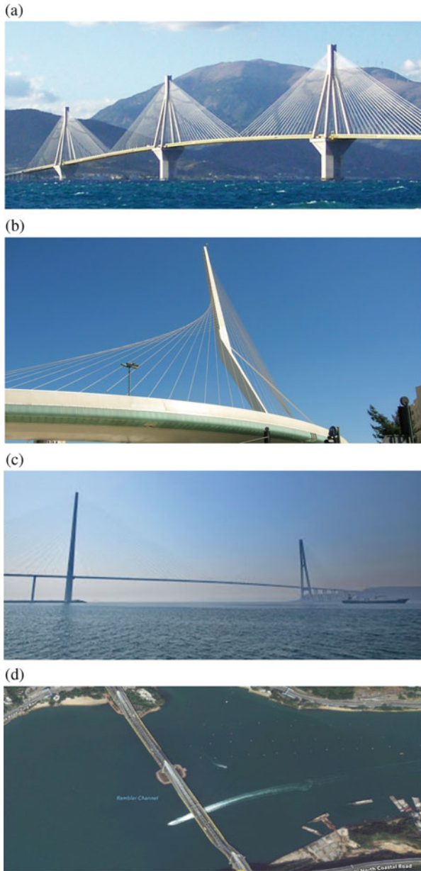
Fig. 1 Cable-stayed bridges all around the world. (a) Rion–Antirion bridge, Greece; (b) Chords bridge, Israel; (c) Russky bridge, Russia; (d) Ting Kau bridge, Hong Kong
