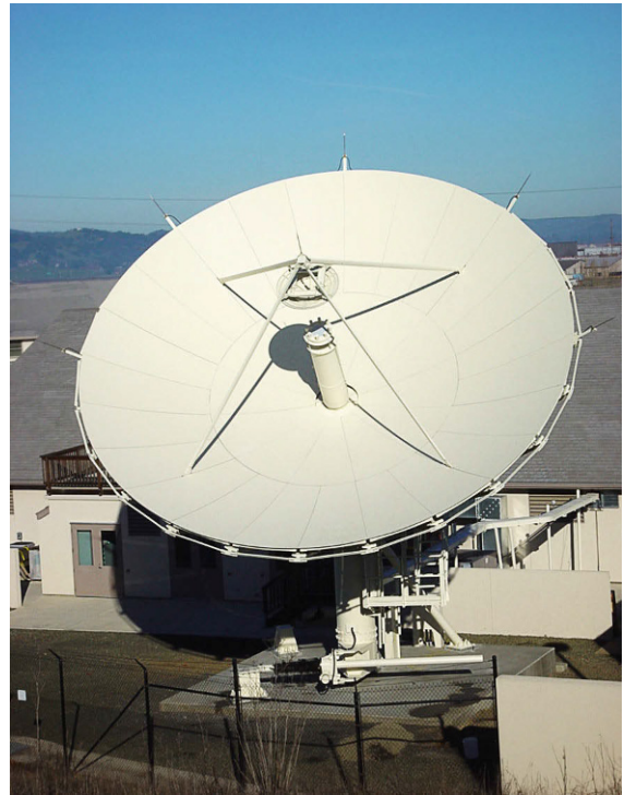
Fig. 12.5 A WAAS geostationary uplink station (reproduced with permission of the FAA satellite navigation team)
