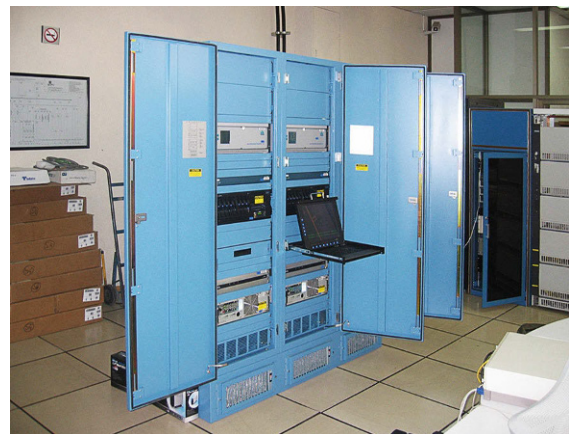
Fig. 12.3 A WAAS reference station (reproduced with permission of the FAA satellite navigation team)
