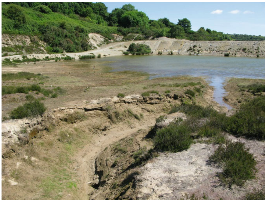
Fig. 1 Granular capping at the upper Wheal Maid tailings lagoon, with evidence of some re-vegetation (foreground) and mine waste used to construct the lagoons (beyond the standing water, middle distance) (color figure online)
