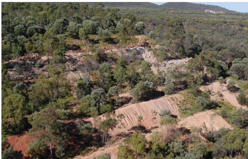
Fig. 3 Aerial photograph of a rehabilitated waste rock dump at a gold mine, northern Australia. An exposed, barren sulfide-rich layer is visible on an outer dump batter. A flawed repository design, inadequate waste characterization and poorly supervised waste management practices led to the exposure of potentially acid-forming (PAF) materials, ineffective encapsulation of PAF materials, physical instability of waste rock batters, erosion, vegetation dieback and impacts on ground and surface waters (color figure online)
