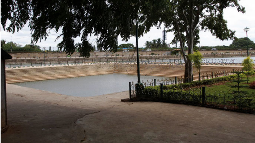
Fig. 3.5 Sankey Tank, one of the many components on Bangalore’s ecological infrastructure. Built in 1882 to meet the water supply demands of Bangalore, restored in the twentieth century as a recreational area (Photograph by Adriana Allen)
