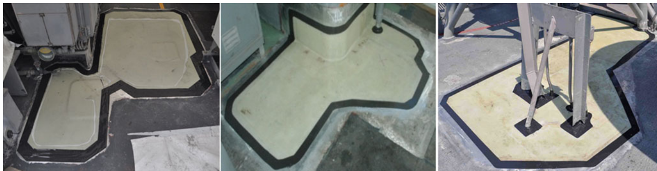
Fig. 3.2 U.S. Navy composite patch repair examples
