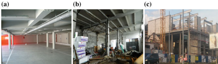
Fig. 1 Examples of the column-beam-plate system: a car park, b storage hall, c building
