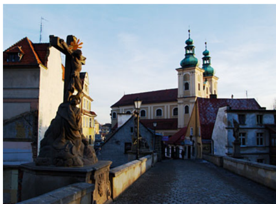
Photograph. 8.8 Kłodzko, the gothic St. John's Bridge (Source M. Stepowicz)
