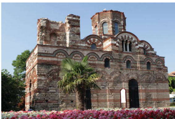
Photograph 3.5 Nesebar— Church of St John Aliturgetos
