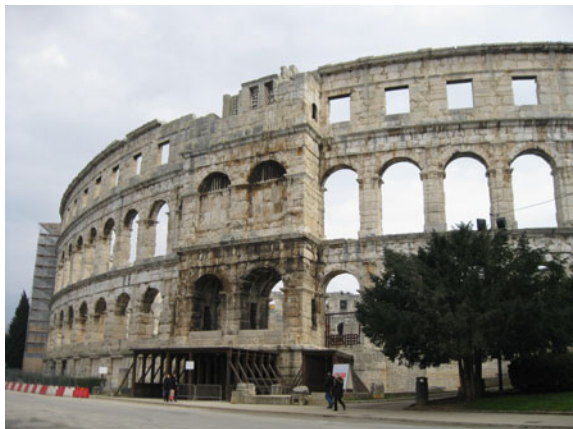
Photograph 4.8 The Arena of Pula—roman amphitheater (Colosseum) from first century AD
