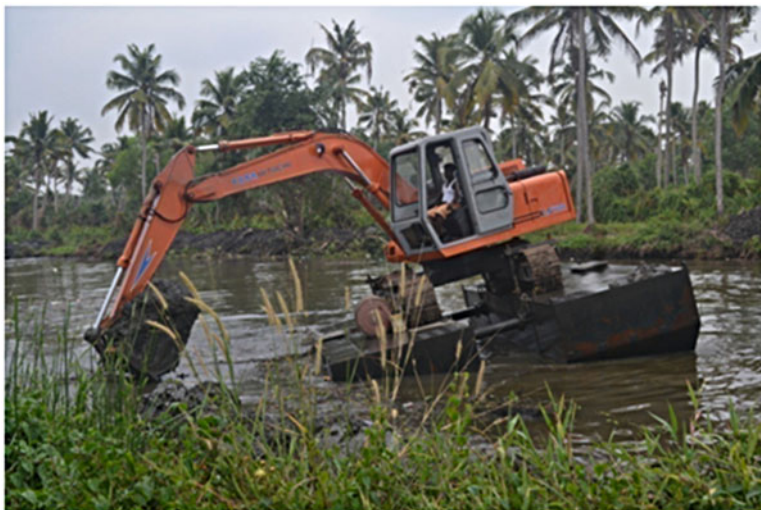
Fig. 10.5 Cleaning of quarry by the BMC of Thrikkakkara Panchayat
