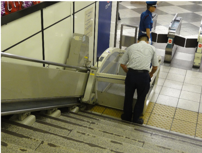
Fig. 4 A Tokyo Metro station some years ago. No elevator was in place, and stair climber was provided. Existing infrastructure makes it difficult to renovate the stairs to introduce elevators more than 10 years passed since the introduction of accessible public transportation law
