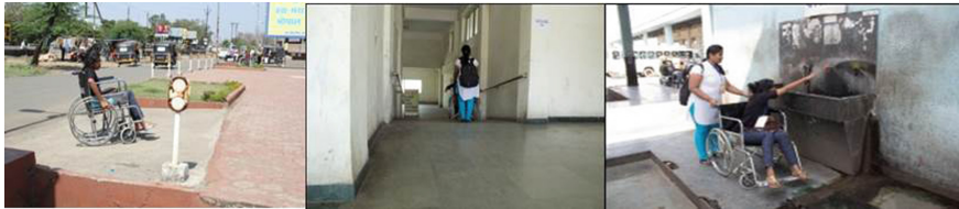
Fig. 9 Identification of problems at Kashubhau Thakre ISBT, Bhopal
