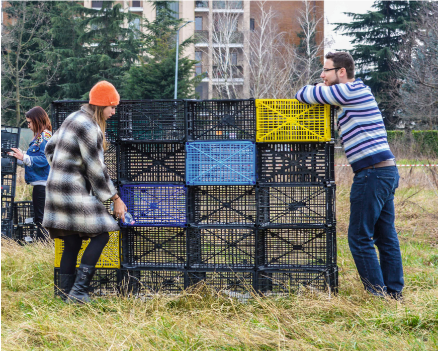
Fig. 4 “Beyond the boundary”, a design activity during “Il Sabato della Bovisasca” to build garden fences by using second-hand plastic crates (used to sell vegetables and fruits) from the local market
