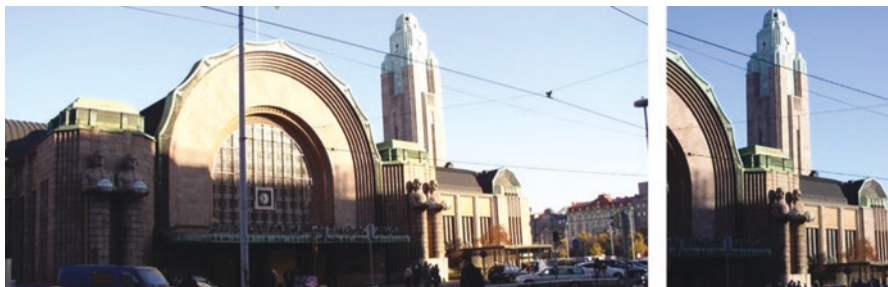
Fig. 1 Helsinki central station (Photo J. Jablonska)
