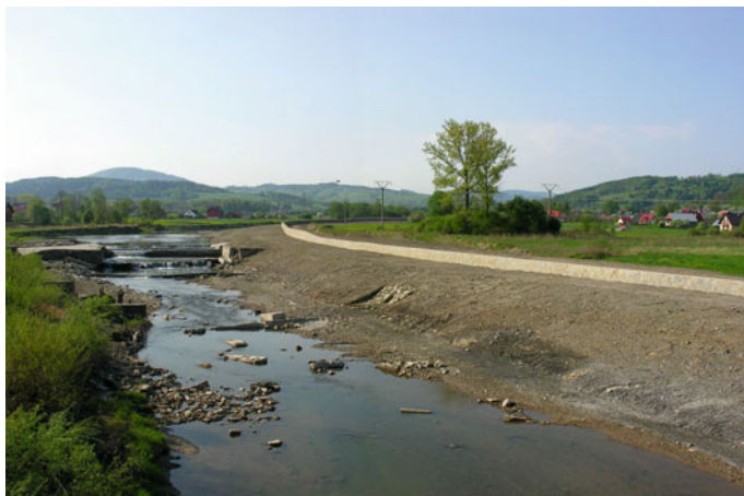
Fig. 3 A concrete wall constructed in 2012 along the Biała River at Stróża under the pretext of preventing the valley floor from flooding. The wall construction resulted in complete eradication of riparian vegetation and separated from the river a wide band of the floodplain that did not require protection from flooding
