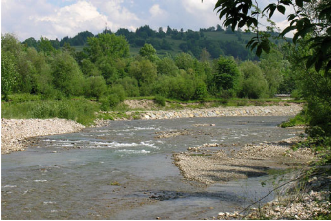
Fig. 2 Rip-rap constructed in 2013 on the concave bank of the Czarny Dunajec at Chochołów protects from erosion a floodplain overgrown with alder and willow shrubs. Buildings that might potentially require protection from erosion are distant from the river bank by more than 100 m, equal to approximately two channel widths at the site
