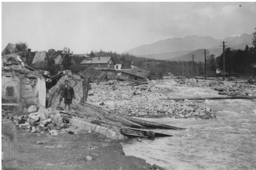
Fig. 1 View of Bystry Stream in its reach within the town of Zakopane just after the catastrophic flood of July 1934. The flood was the largest one on record in this region, with peak discharges of streams flowing from the Tatra Mountains up to three times higher than the largest ones recorded in the second half of the 20th century. Visible are destroyed houses in the riparian area and huge amounts of coarse bed material deposited practically at the level of the developed valley floor. Currently the stream flows in 6 m-wide, stone-lined, artificial channel. The photo no. 1-G-4647-12 of the National Digital Archive of Poland
