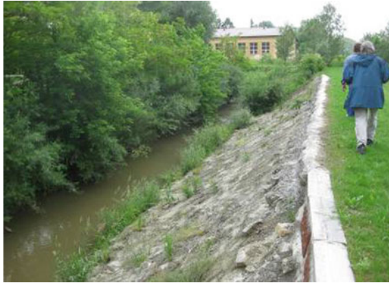
Fig. 1 Reinforced stream bank. Source Małgorzata Siudak
