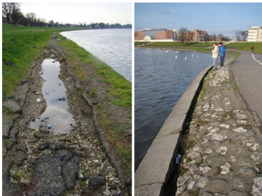
Fig. 6 Destruction of the low boulevard of the River Vistula in the vicinity of the Dębnicki Bridge, in Cracow, resulting of the 2010 flood. Self Source (Politechnika Krakowska)
