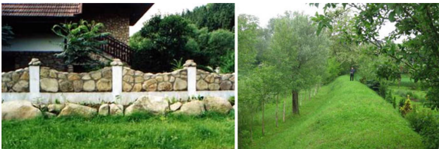
Fig. 3 Examples of a stone wall and an earth dike, protecting houses. Source Małgorzata Siudak, Roman Konieczny
