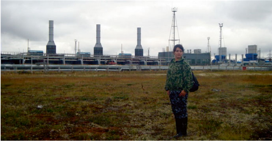
Fig. 1 View of unit-2 from North to South
