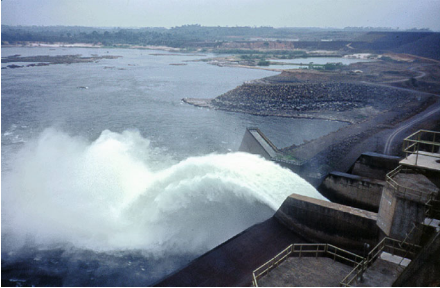
Fig. 6.1 Spillway of the Tucuruí Dam in the Tocantins River, state of Pará. Water leaves the reservoir at a depth of 20 m, where it carried great quantities of methane. Pulverization in the form of droplets releases this greenhouse gas in the atmosphere, contributing to global warming (photograph by Philip M. Fearnside)
