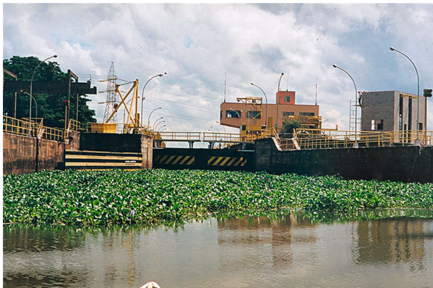
Fig. 11.2 Eutrophication of reservoirs such as the Barra Bonita Dam can interfere in the functioning of locks and turbines. Photograph: J. G. Tundisi
