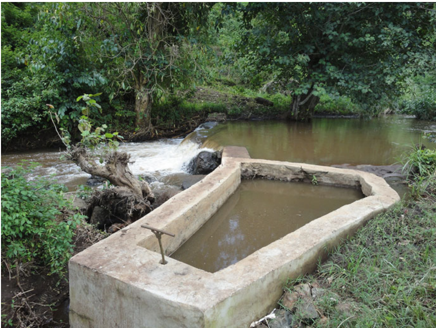
Fig. 7 Gravity water scheme at Sanzara Parish after completion (Photo by IUCN – Uganda)
