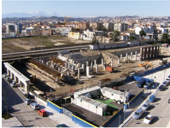
Fig. 2 Redevelopment of Pescara Porta Nuova railway station, 2008
