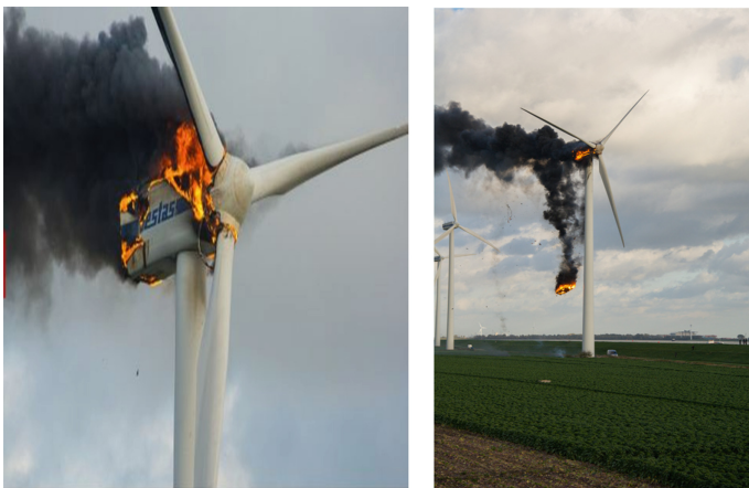
Fig. 2. Fire in wind turbine
