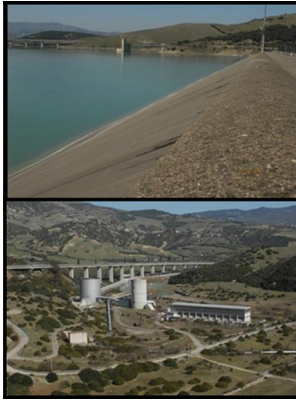
(a) Monte Cotugno dam: one of eight dams managed by EIPLI.
