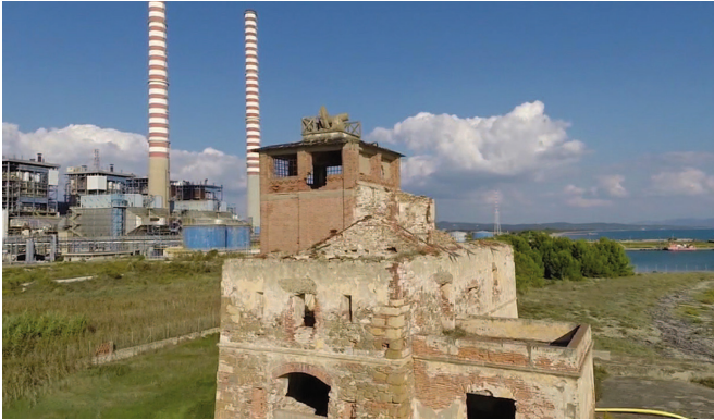
Fig. 2. The Torre del Sale, with the ENEL power plant in the background, and beach to the right
