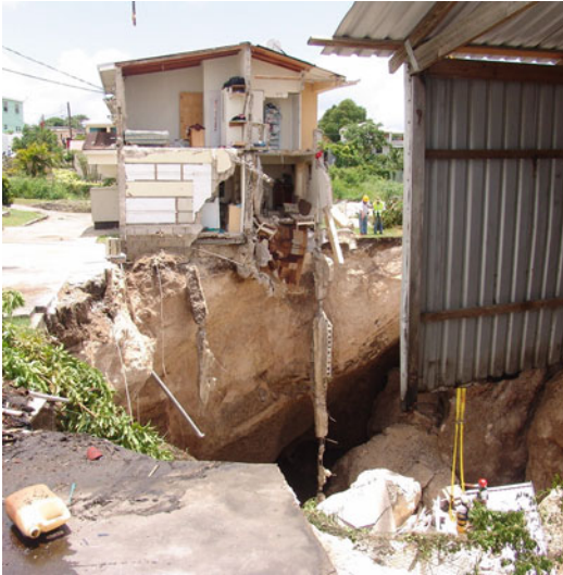
Fig. 32.19 Sinkhole in Barbados 2007 killing a family of five presenting a hazardous working environment (Copyright: Authors' own image)
