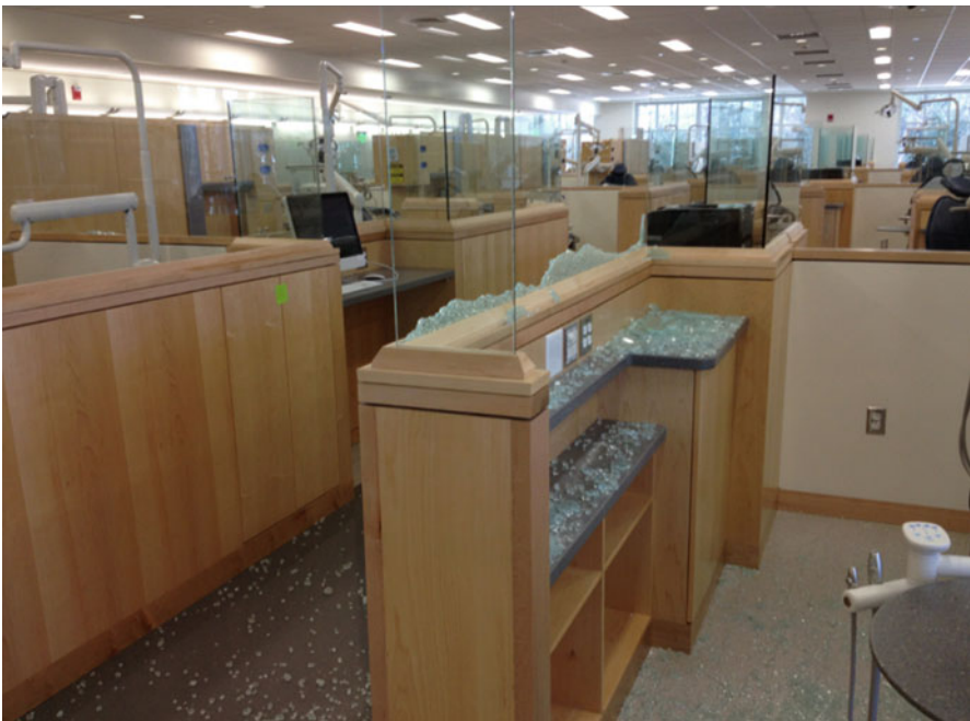
Fig. 26.6 Comprehensive Care clinic operatories at ECU, showing early shattering of glass dividers
