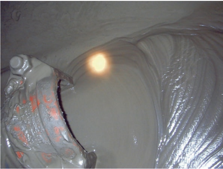
Fig. 11.10 Backfill slurry discharge
