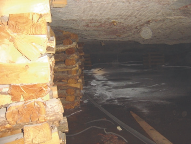
Fig. 11.14 Backfill in panel 416
