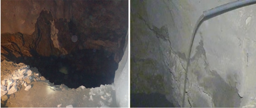
Fig. 5.19 Photos of the typically paste backfill placements to underground open stopes
