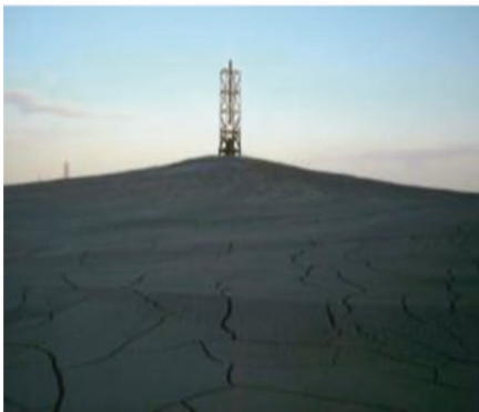
Paste deposition forming a cone around a deposition tower
