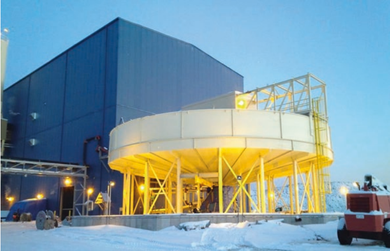
Fig. 12.6 22 m diameter high-rate thickener—bolted tank construction. This thickener receives tailings from the mill and dewateres the slurry to about 70 wt% solids
