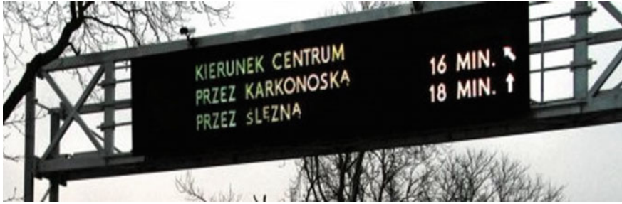
Fig. 2 An example of a variable message board in the city of Wrocław. Two travel times are displayed for the direction: City centre, via: Karkonoska St., and via: Ślężna St.
