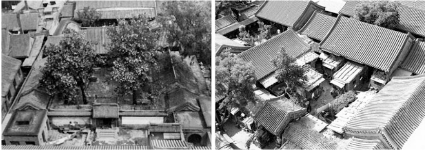
Fig. 4.11 An original courtyard house in the 1950s ( left ), and courtyards with many additions in 1980s ( right ). Source By courtesy of the Reference Room of the School of Architecture, Tsinghua University
