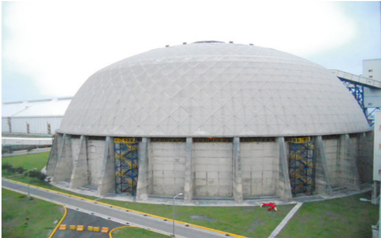
Fig. 1.10 Dome indoor yard-exterior
