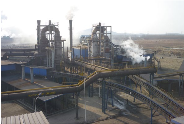
Fig. 7.2 A rotary hearth furnace plant in Shandong Province, China
