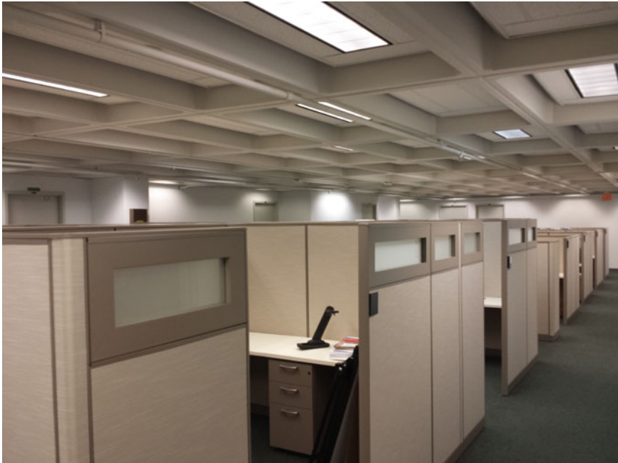
Fig. 1.6 Core zone of a large office building lacking access to daylight and views. A homogeneous and steady-state lighting condition is provided by ambient overhead fluorescent lighting. In such environments, lighting provided by electrical sources may be adequate for visual task performance but lack the appropriate spectrum and intensity required to effectively stimulate the circadian system, creating zones of “biological darkness”
