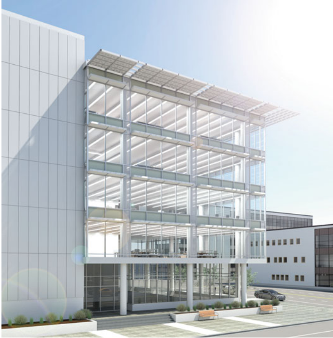
Fig. 3.47 Rendered (conceptual) view of building facade and interior ceilings showing daylight delivered from SunLuminaire™ fixtures. Image credit SunCentral
