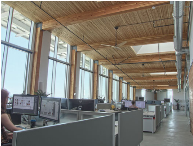
Fig. 2.4 Sixth floor daylit perimeter zone. Note the absence of a conventional installation of electrical lighting fixtures on the ceiling
