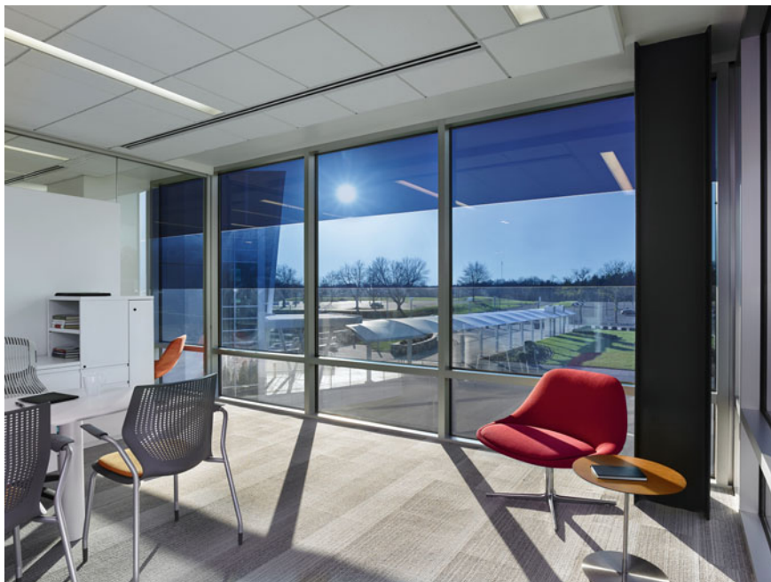
Fig. 3.41 Facade glazed with EC units subdivided vertically. Tint state of horizontal groups can be independently adjusted to improve glare control while preserving clear views to the outdoors. Image Credit Sage Glass, LLC
