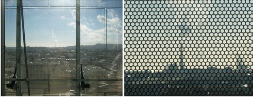
Fig. 2.46 Interior views looking through the facade glazing and exterior perforated metal screen at distances of 1 m ( left ) and 0.1 m ( right )
