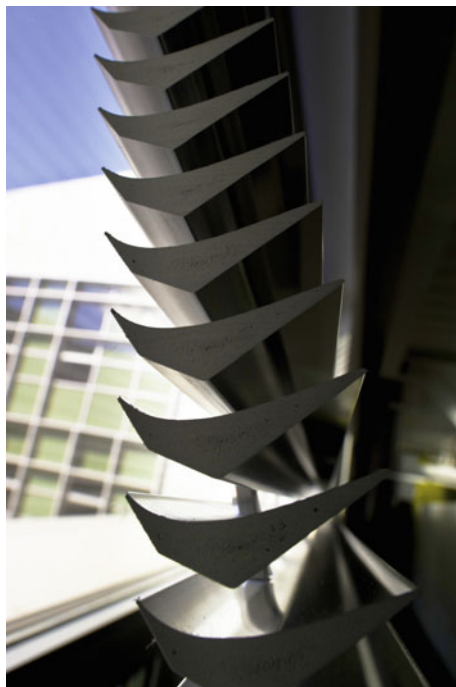
Fig. 3.5 Close up profile view of a LightLouver™ daylighting system unit during installation. After installation the unit is parallel to the window glazing (inboard side). The LightLouver™ daylighting system units redirect sunlight deeper into the office space to reflect off ceilings and provide ambient lighting. Image credit Dennis Schroeder/NREL
