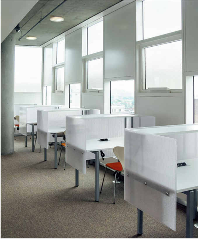
Fig. 5.11 The alternating pattern of window penetrations is integrated with the internal programming of the library perimeter zone. Image credit Behnisch Architekten
