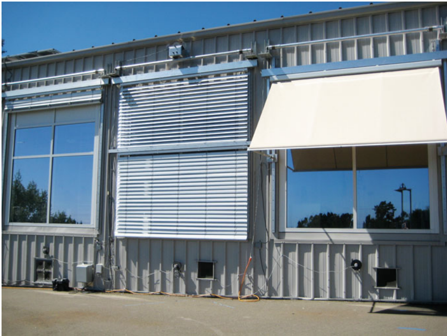
Fig. 4.31 LBNL windows testbed facility (south-facing facade) showing comparison of two exterior shading systems to an unshaded window reference case
