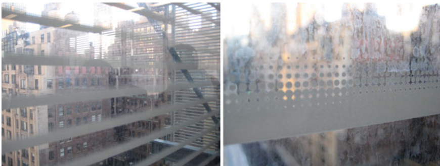
Fig. 2.49 Horizontal frit pattern applied to portions of the glazed facade of New York Times building
