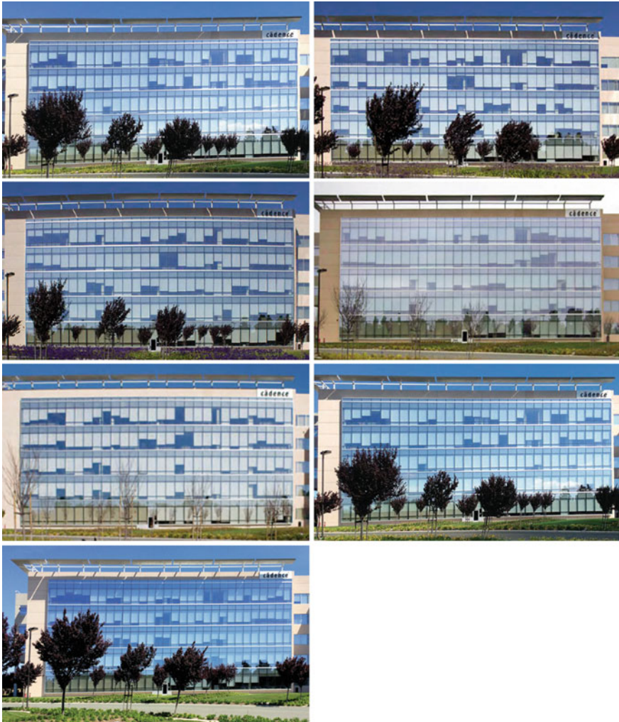
Fig. 1.10 Example operational outcome for a “transparent” facade located in San Jose, California, a climate with predominantly clear skies. Date of each image, clockwise from top left, August 2009, December 2009, January 2011, October 2012, April 2014, August 2011, August 2010. Image credit Prof. Charles Benton
