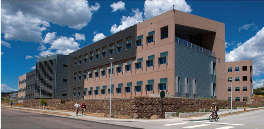
Fig. 5.18 The National Renewable Laboratory (NREL) Research Support Facility (RSF), south facade. Exterior vertical metal panels attached to opaque sections of the facade operate as a transpired solar collector to passively pre-heat ventilation air during the heating season. This image has been reprinted with permission from National Renewable Energy Laboratory
