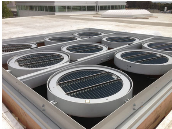
Fig. 3.44 Exterior view of the SunCentral SunBeamer™ installed in a skylight configuration. Image credit SunCentral
