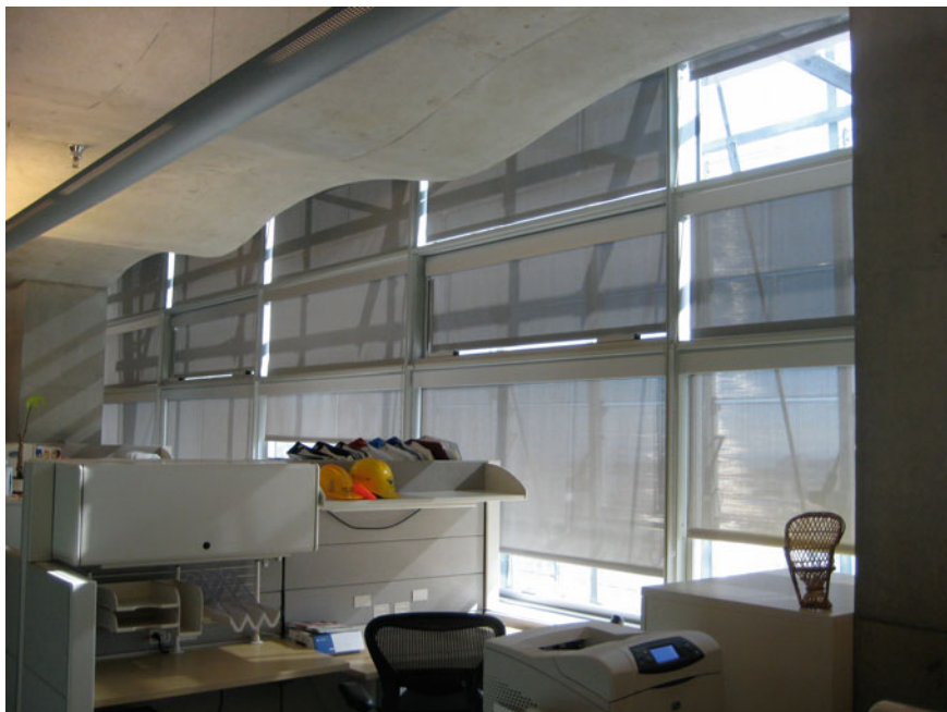
Fig. 4.20 Interior roller shades deployed in perimeter zone of daylight office building, limiting daylight transmission and views, and leading to the use of electrical ambient lighting adjacent to windows during daytime
