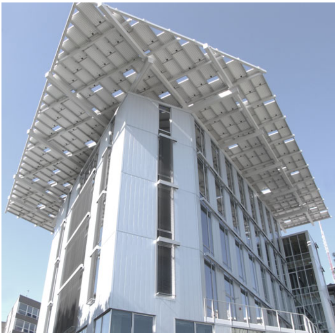
Fig. 5.28 Exterior view of the Bullitt Center from street level showing exterior shading deployed on facade in direct sun and exterior shading retracted for facade in shade
