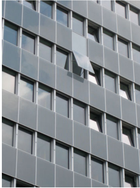
Fig. 3.35 Dynamic facade applied as a retrofit in 2005 to the Kreditanstalt für Wiederaufbau (KfW) building located in Frankfurt Germany, originally built in 1968. The facade incorporates dual-pivot manually operable windows for natural ventilation, which are dynamically shaded by automated exterior sunshades that retract into the spandrel zone of the facade when not required
