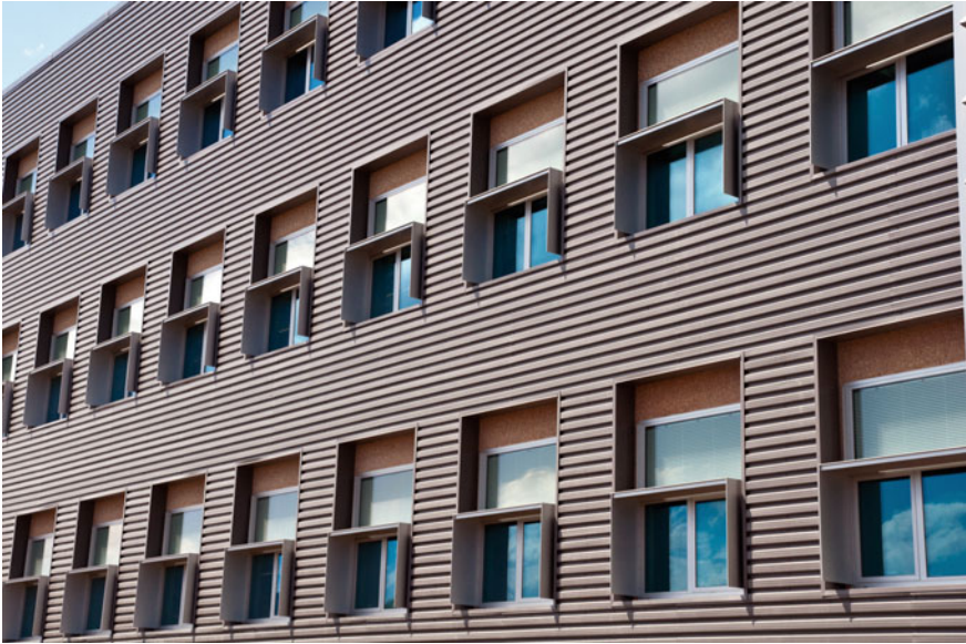
Fig. 3.8 NREL RSF south elevation showing functionally subdivided windows. Image credit Pat Corkery/NREL
