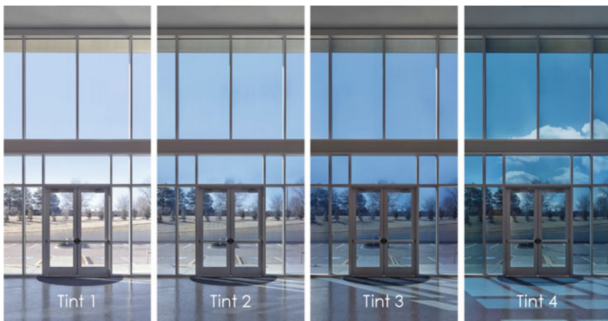
Fig. 3.40 Transition in EC tint state from fully clear ( left ), to fully darkened ( right ). Optical properties for each state are (Tint 1: VLT = 0.58, SHGC = 0.46; Tint 2: VLT = 0.40, SHGC = 0.29; Tint 3: VLT = 0.20, SHGC = 0.16, Tint 4: VLT = 0.03, SHGC = 0.09). Image credit View Glass, LLC
