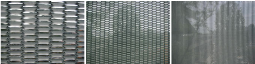
Fig. 2.48 The Haupthaus exterior solar control screens are composed of a glazed sandwich panel with an interlayer of expanded metal configured to completely block direct view of the solar disc from the interior while preserving a partial view to the exterior. Images are taken from the building interior at varying distances from the screen (0.2, 1, and 3 m)
