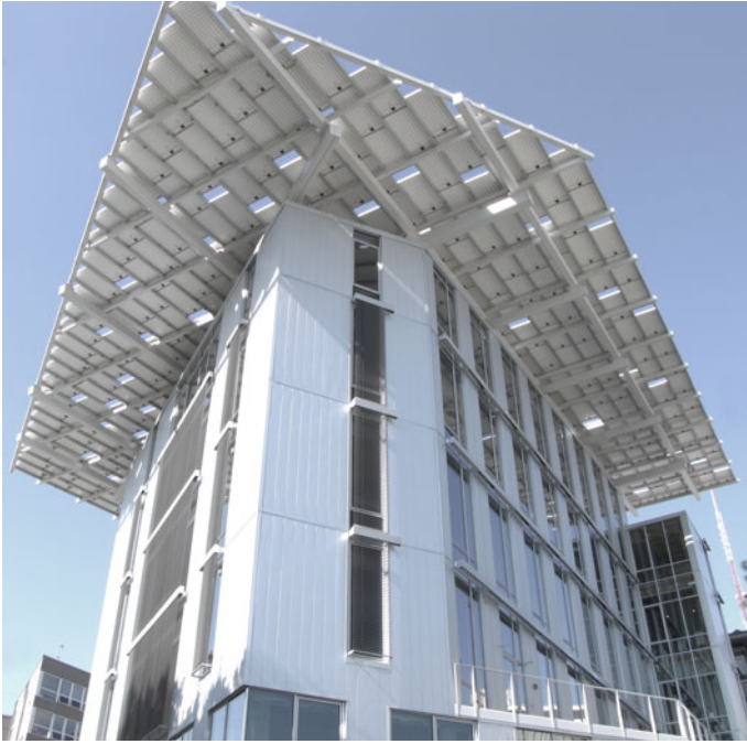
Fig. 2.3 Exterior view of the Bullitt Center showing rooftop solar PV array and exterior automated shading devices
