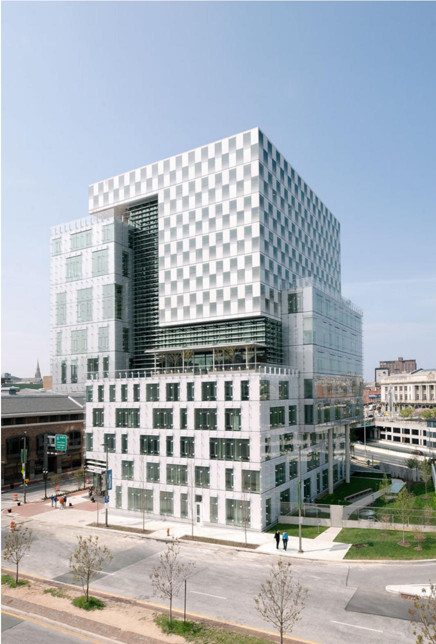
Fig. 5.1 Exterior view showing three facade types (office/classroom, library, and atrium). Image credit David Matthiessen, David Matthiessen Photography
