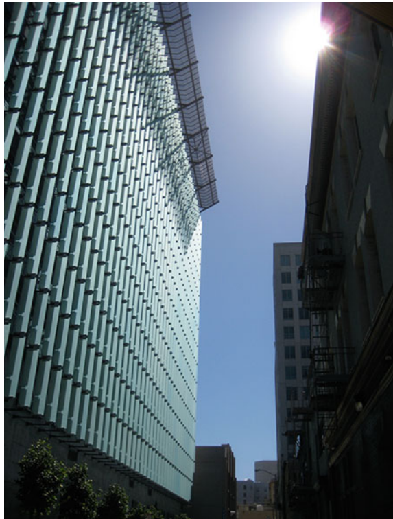
Fig. 2.26 Exterior view of translucent vertical louvers shown in Fig. 2.25
