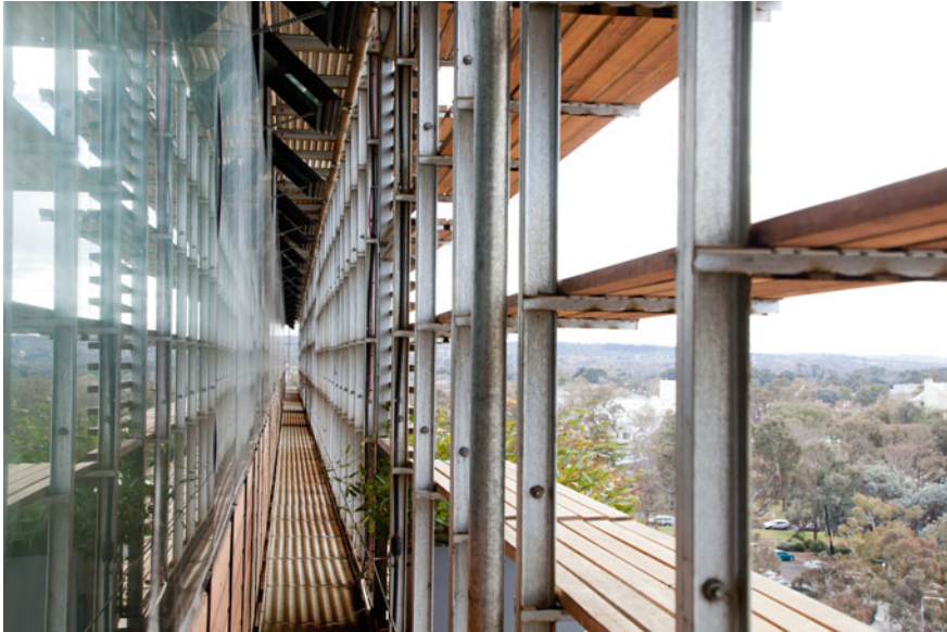
Fig. 1.13 View along integrated access way showing open state of automated upper windows . Image credit Carl Drury
