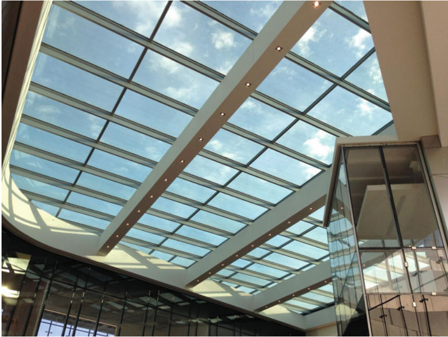
Fig. 3.42 Image of 255 m 2 ceiling skylight of the Connor Group headquarters in Dayton Ohio, glazed with View Glass, LLC. The EC glass switches from clear (as shown) through several tint levels based on the sun’s position in the sky. Image Credit View Glass, LLC
