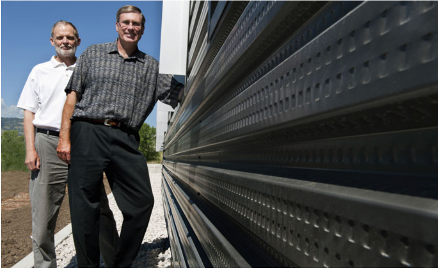
Fig. 5.23 Transpired solar collector installed on south facade of the RSF. Image credit Dennis Schroeder, NREL
