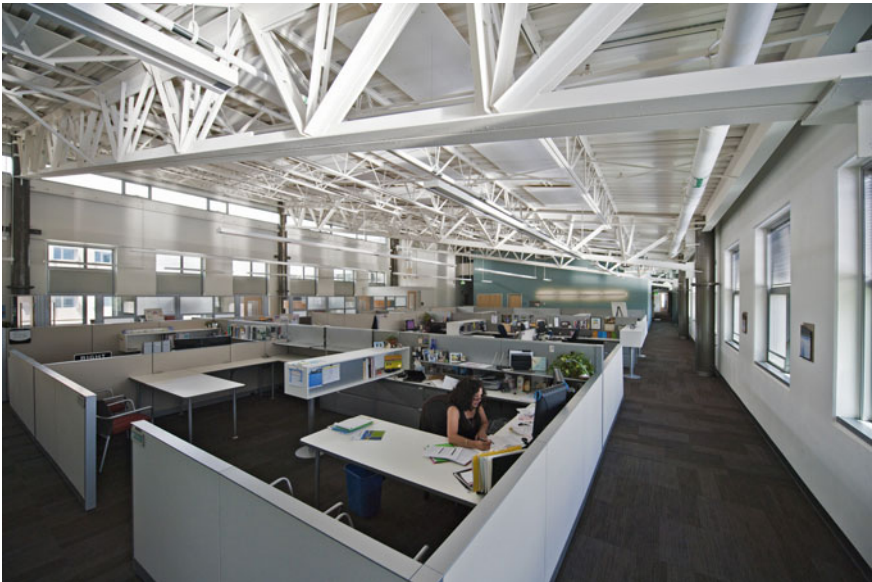
Fig. 3.9 The LightLouver™ daylighting system units installed in the daylight windows ( right side of image ) redirect sunlight deep into the office space to provide ambient lighting. Image credit Dennis Schroeder/NREL
