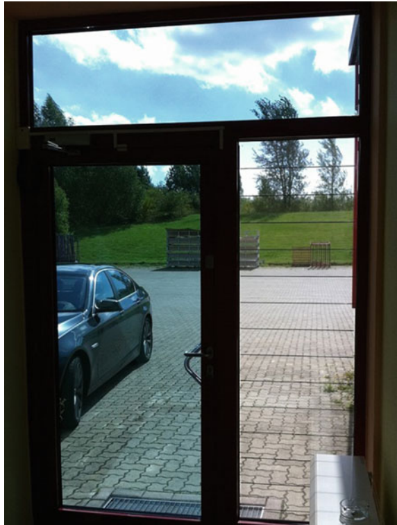
Fig. 3.13 Comparison of view to outdoors looking through MicroShade™ (installed in right window ) versus solar control glass ( door and top window ). Image credit MicroShade
