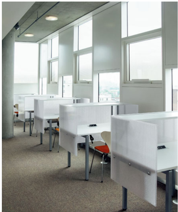
Fig. 3.25 Interior view of the library facade of the John and Frances Angelos Law Center showing alternating window pattern, where the application of frit preserves both views downward near desks and clear views to the sky from upper window regions. Image credit Behnisch Architekten
