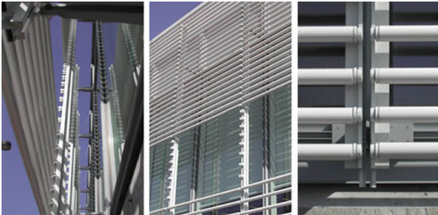
Fig. 5.35 Exterior facade of daylighting mockup. Photographs by: Voropat Inkarojrit. Image credit LBNL
